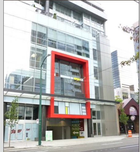
Figure 18: Access to below grade parking is discretely executed at grade without compromise to the pedestrian environment or manner in which the building relates to the street.
